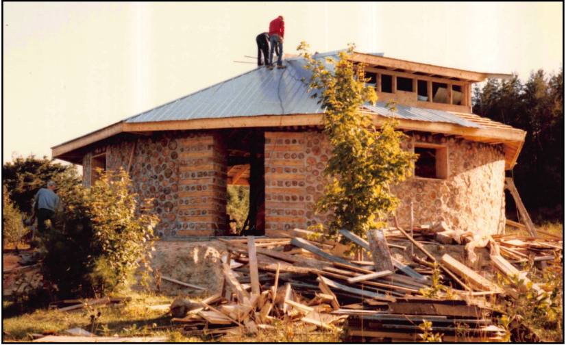
Figure 54: Installing the roof on the cordwood house, September 1985
