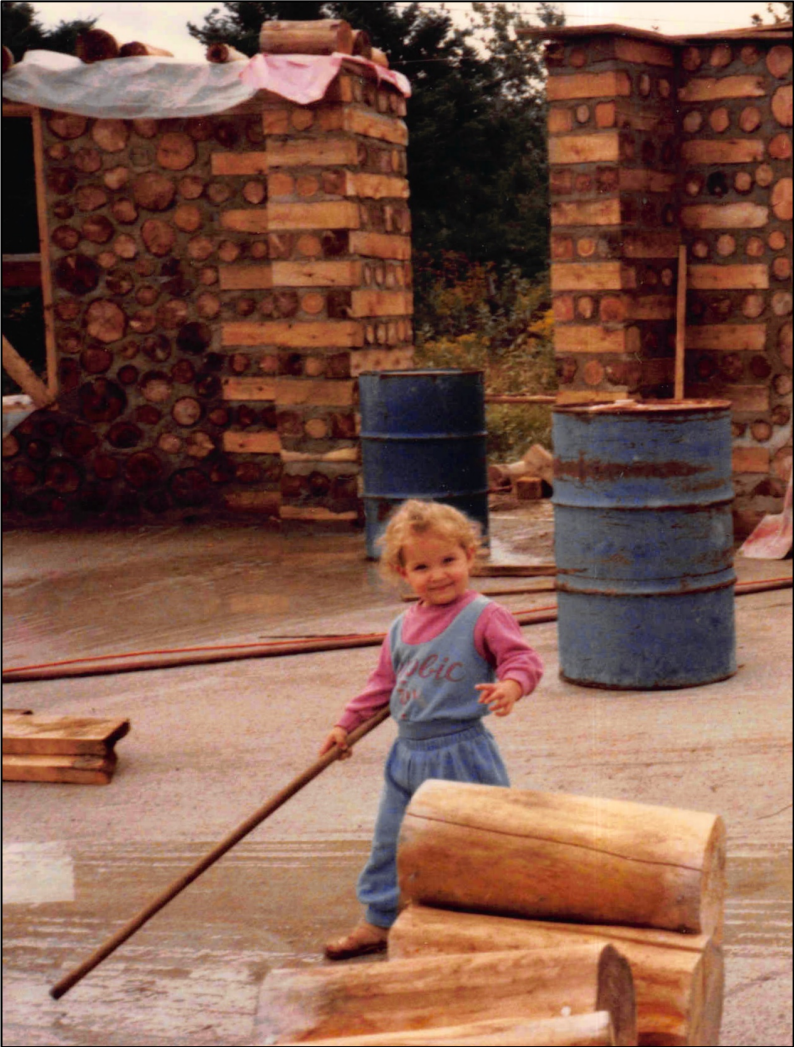
Figure 53: Esther, almost 3, playing on the foundation of the round house, 1985.
